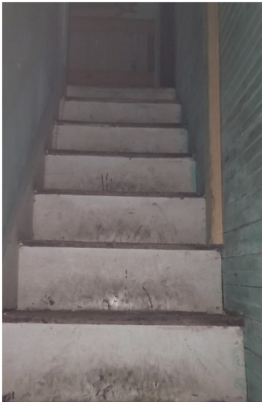
Stairs from first floor (2024)
