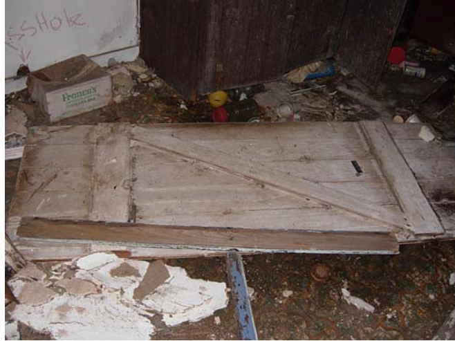
Interior plans door in northwest room
