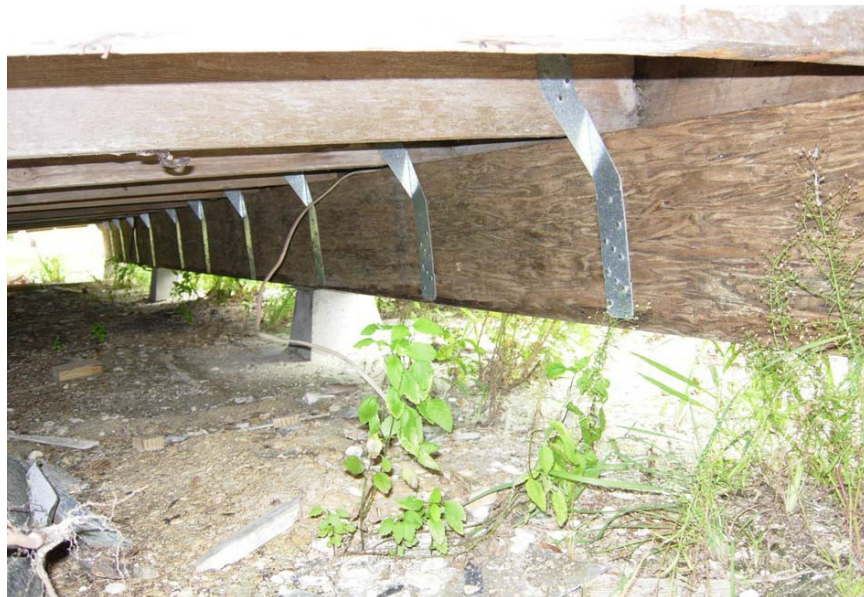
Floor joists on new foundation system with galvanized connectors (2008)
