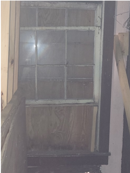
Second Floor East window typical 6/6 sash (2024)
