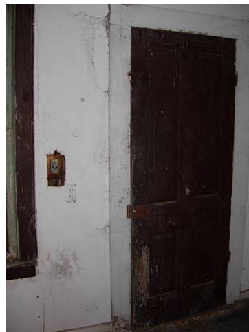
Interior view of north door, west end
