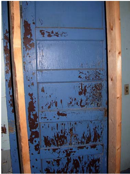
Interior view of south (front) door
