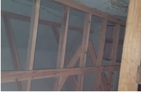
Loft west side, shoring and diagonal braces (2024)
