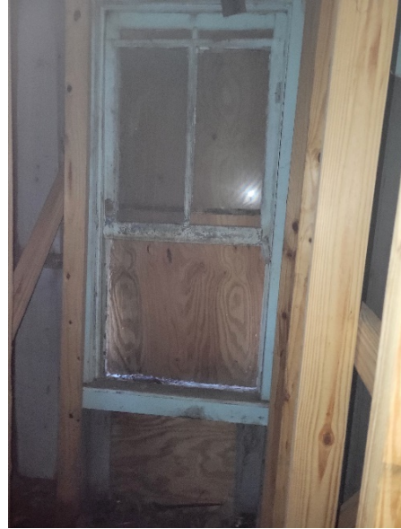
Second floor North window 2/2 sash at east dormer (2024)
