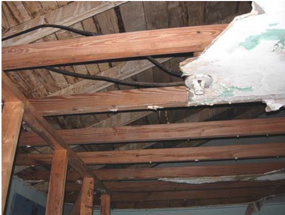
Roof rafters at shed roof section with later ceiling joists and tongue and groove roof deck (2008)
