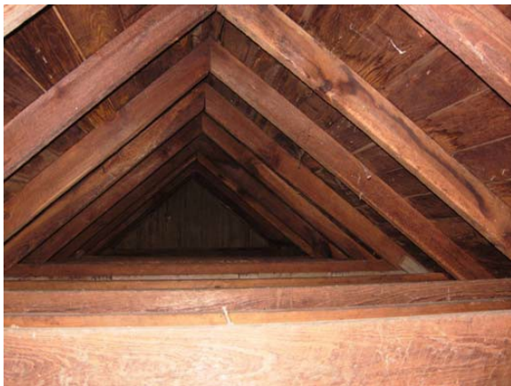
Attic rafters and collar ties (2008)
