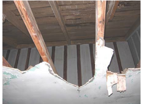
Roof rafters at shed roof section with later ceiling joists and tongue and groove roof deck (2008)
