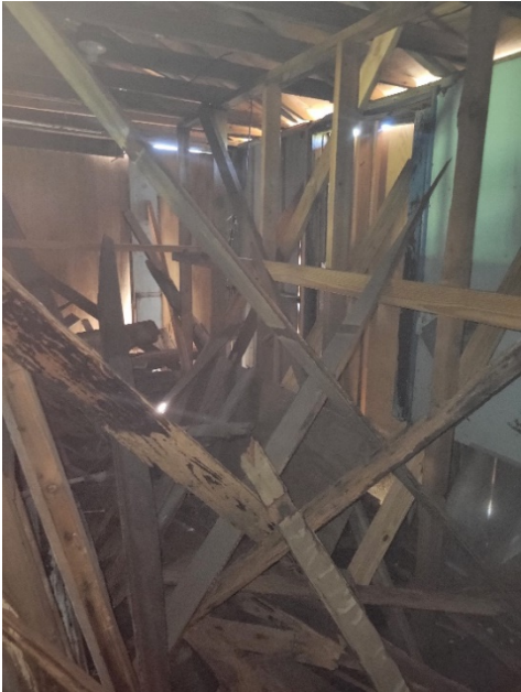
Ceiling framing and roof rafters south room looking east (2024)
