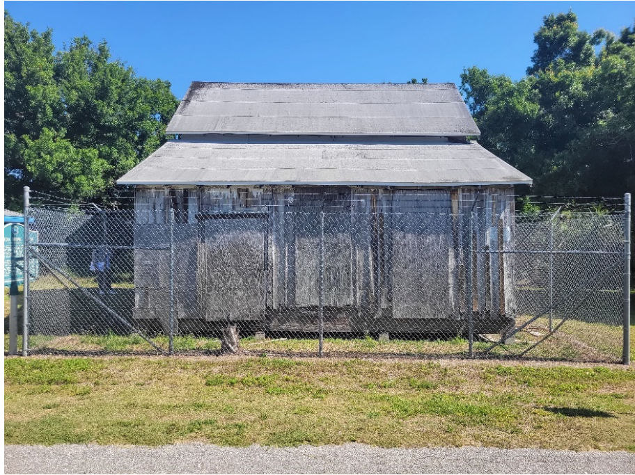
Facade: South Elevation (2024) facing access road to Cape Haze Pioneer Trail
