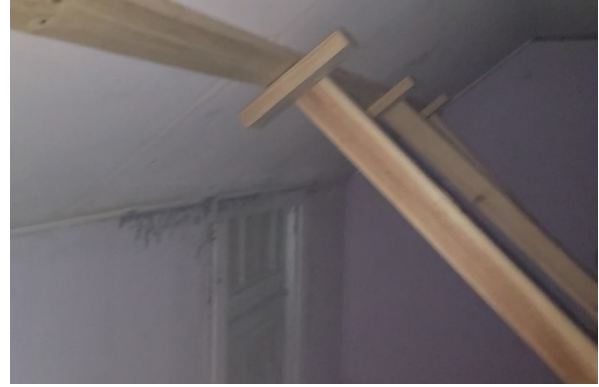
Loft east side, shoring and diagonal braces
