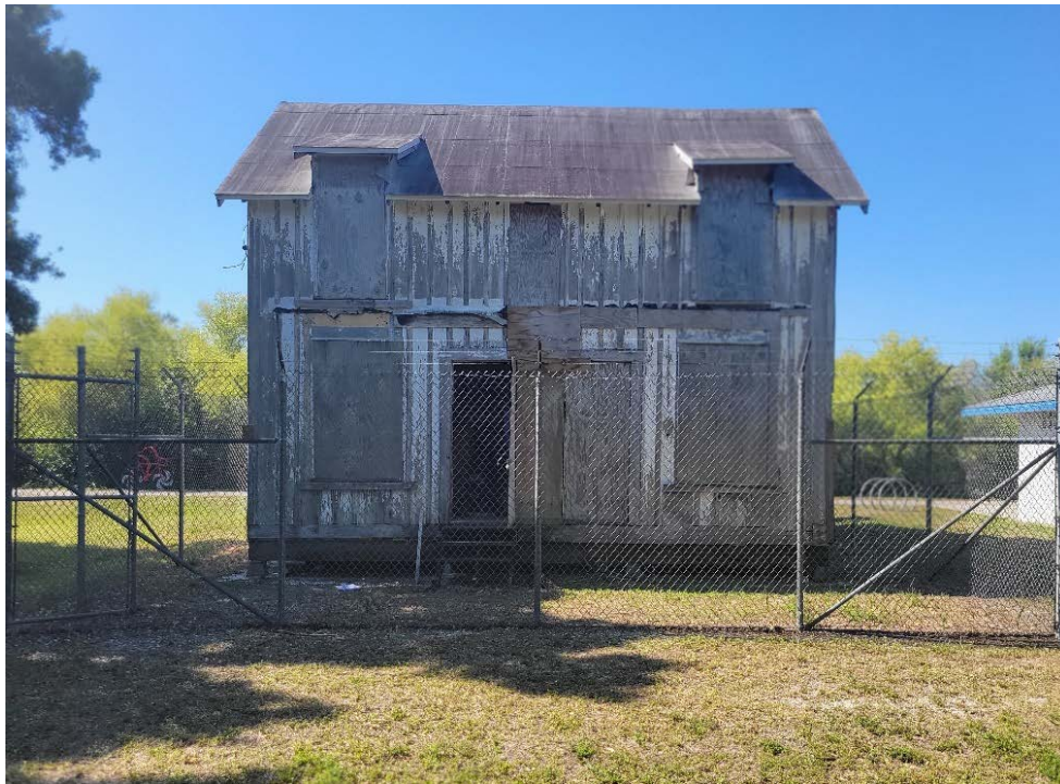
Facade: North Elevation (2024)
