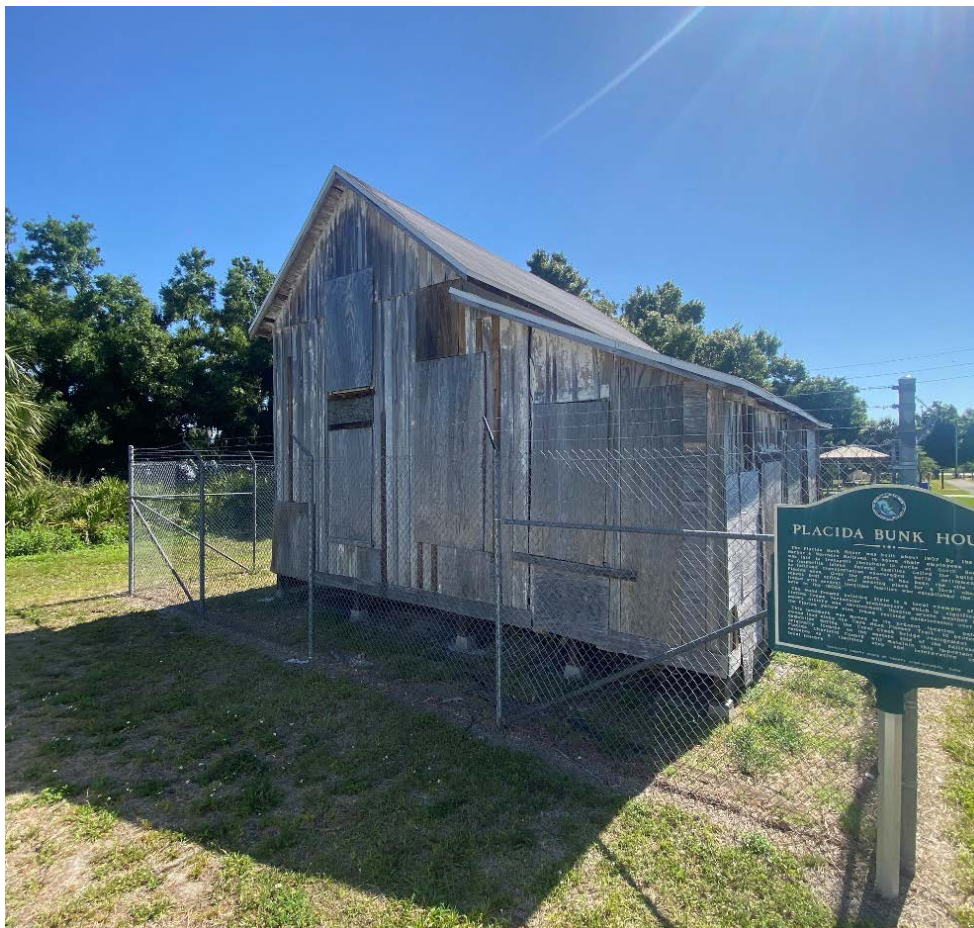
Facade: West Elevation (2024)
