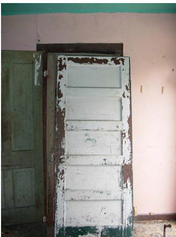
Interior view of north (rear) door on east end
