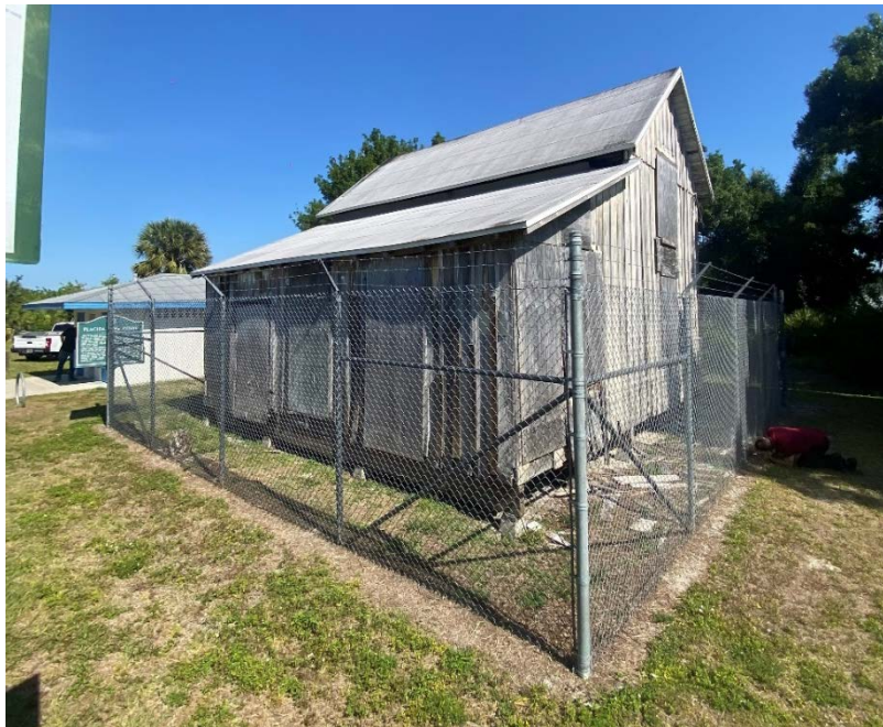
View of southeast corner, with roof covering in fair condition. (2024)
