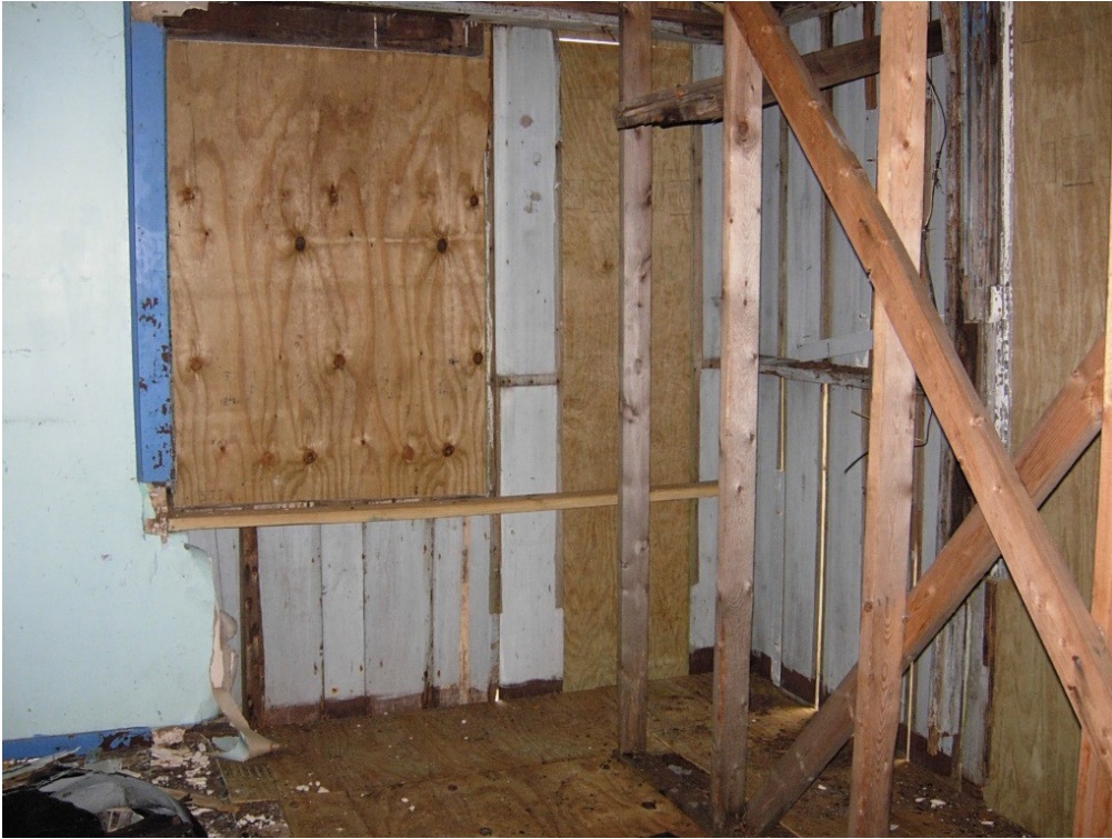
East wall of south room with wallboard removed (2008)
