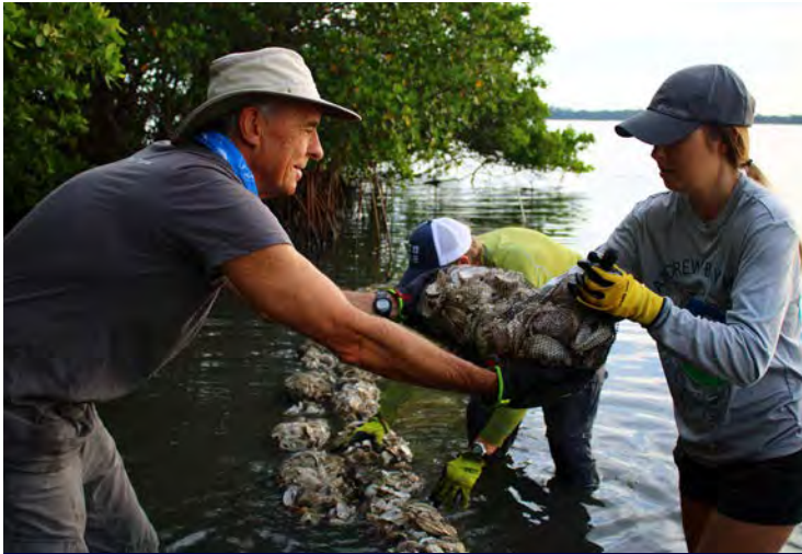
Ecosphere Restoration founder Tom Ries installing oyster reef materials as part of hands-on living shoreline restoration to enhance coastal habitat and resilience
