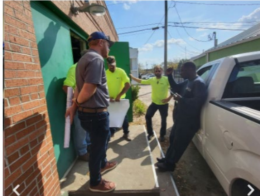
Flovac personnel and City staff at Vacuum Sewer Collection Station.
