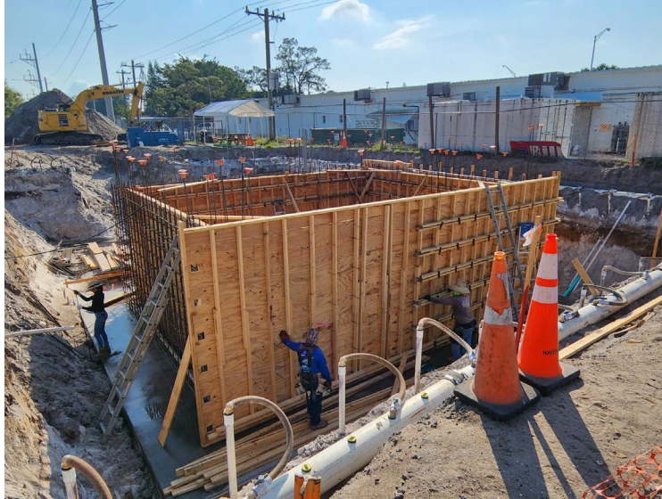
Figure 3 Flovac Vacuum station dry well form work
