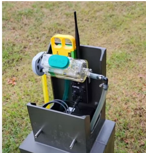
Figure 20 Flovac Air Terminal housing valve controller and monitoring
