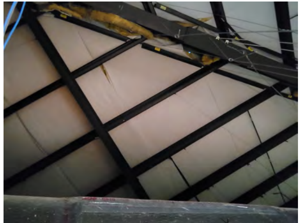
Figure 31: Insulation visible near roof ridge.
