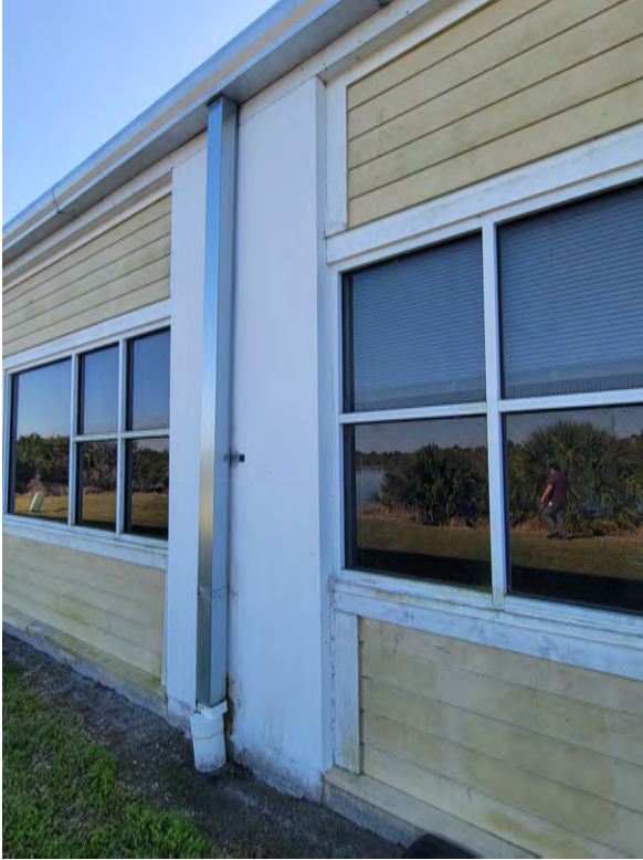
Figure 14: Rear wall at north end of building.
