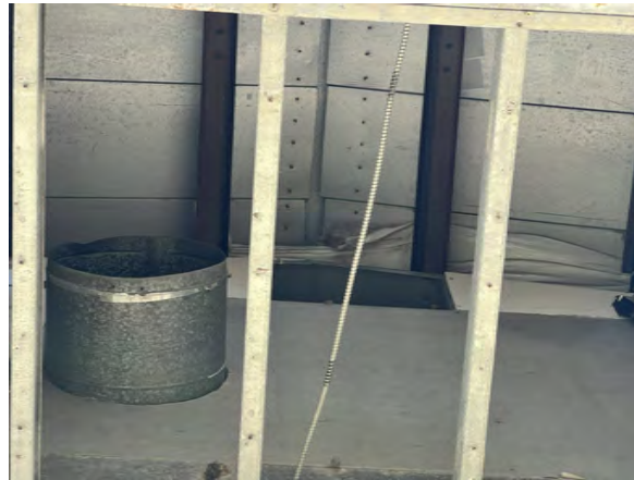
Figure 9: Duct visible inside structure.
