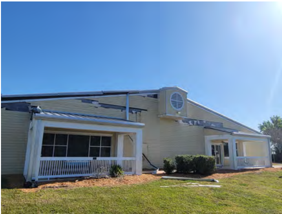
Figure 4: General condition of East Port Environmental Campus exterior.
