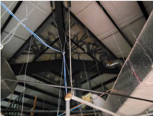
Figure 30: Roof ridge visible through attic space.
