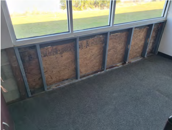
Figure 20: Exposed wall studs and sheathing.
