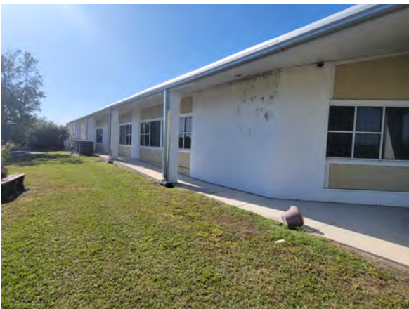
Figure 12: Rear wall at north end of building.
