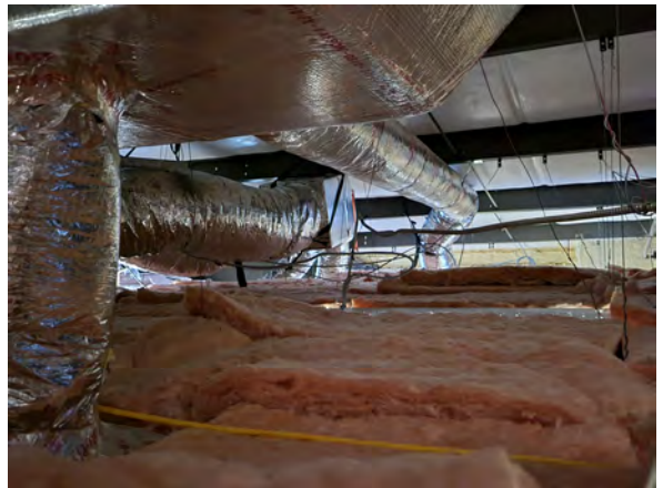
Figure 27: Attic space above ceiling stains showing HVAC ducting.
