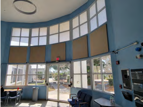
Figure 16: Interior view of lobby, full height glazing visible.
