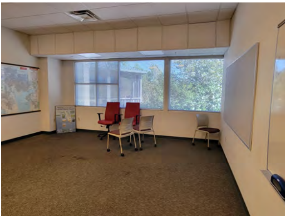
Figure 18: Training room interior condition.
