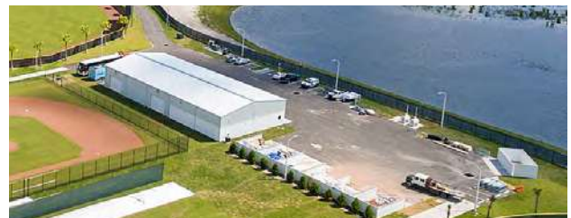
Atlanta Braves Cool Today Park | Maintenance Facility
