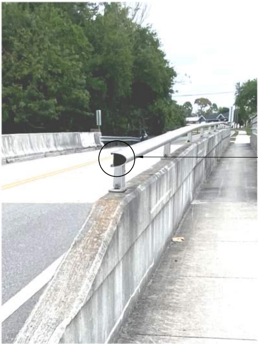
BULLET RAILING END CAP DETAIL
