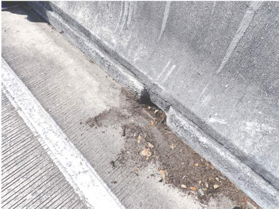
Existing Deck Drain (To be cleaned)
