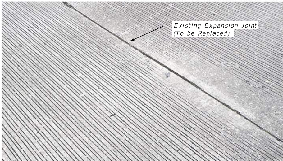
Bridge Expansion Joint (Other Expansion Joints similar)
