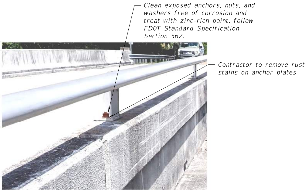
TYPICAL BULLET RAILING ANCHOR CLEANING DETAIL
