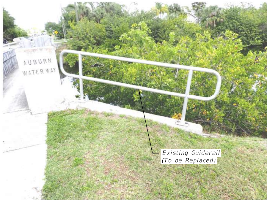
Existing Guiderail (Southeast Wingwall guiderail shown)
