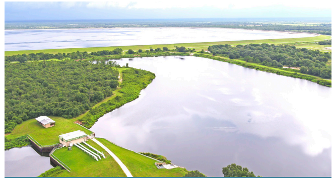
Peace River Reservoir No. 3 expansion featured watershed-scale hydrologic modeling and conveyance design. We will apply this experience to this project.
