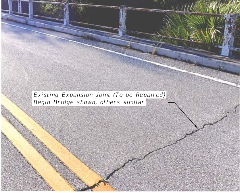
Bridge Expansion Joint
