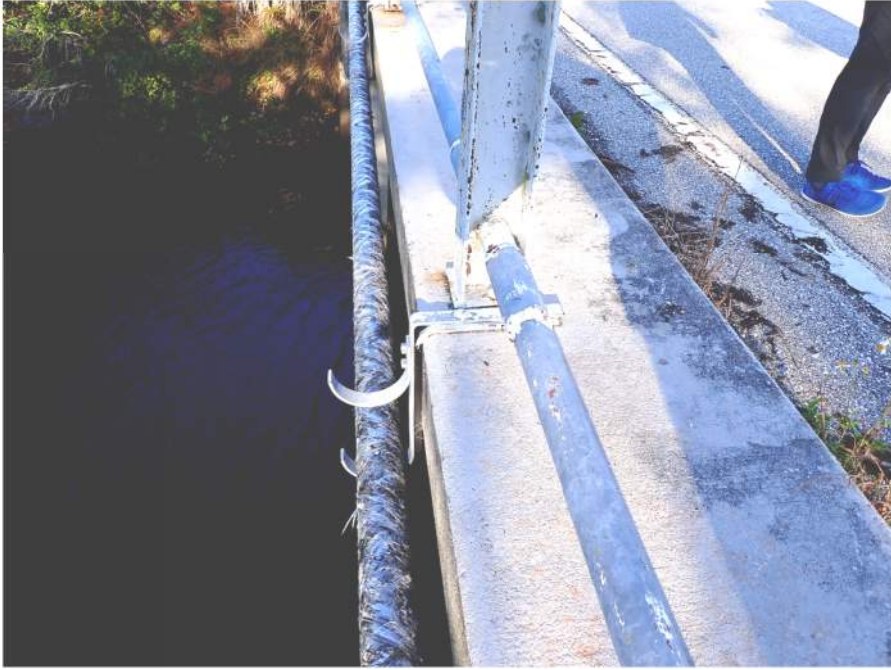
Existing Utility Hangers (To be Replaced)
