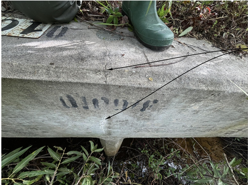
PHOTO 5 - RIGHT HEADWALL OVER WALL 2
