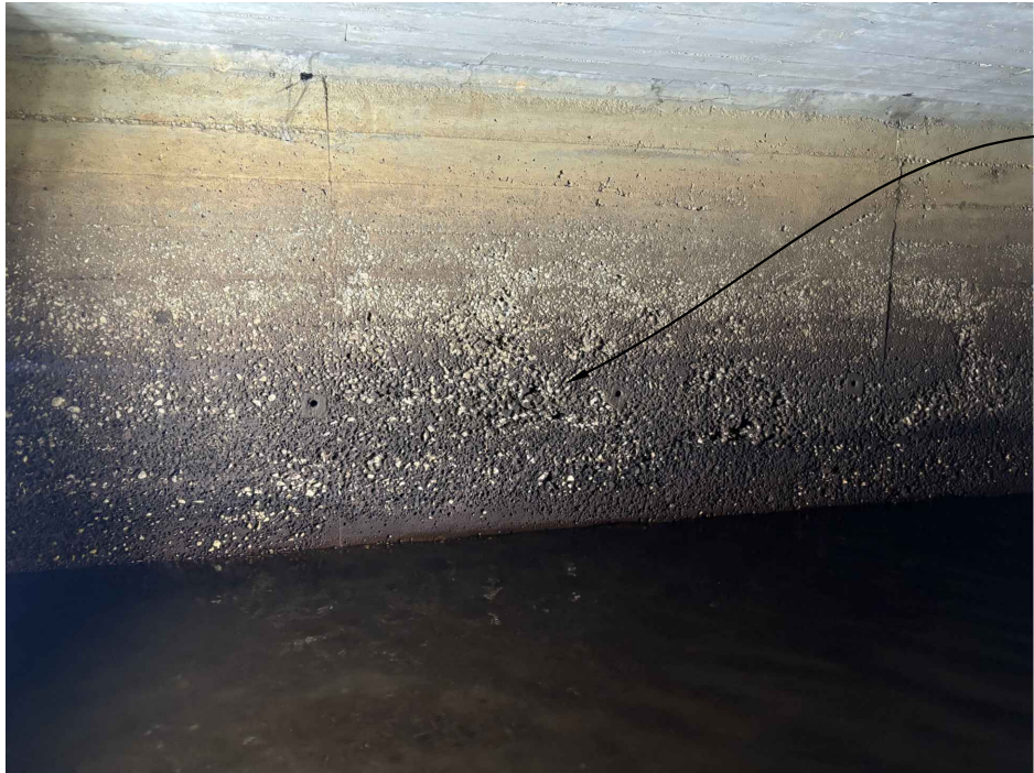
PHOTO 7 - TYPICAL SIDE WALLS
