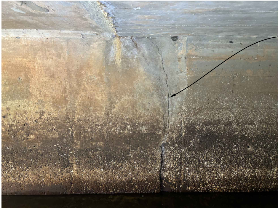
PHOTO 11 - TYPICAL AT WIDENING JOINTS
