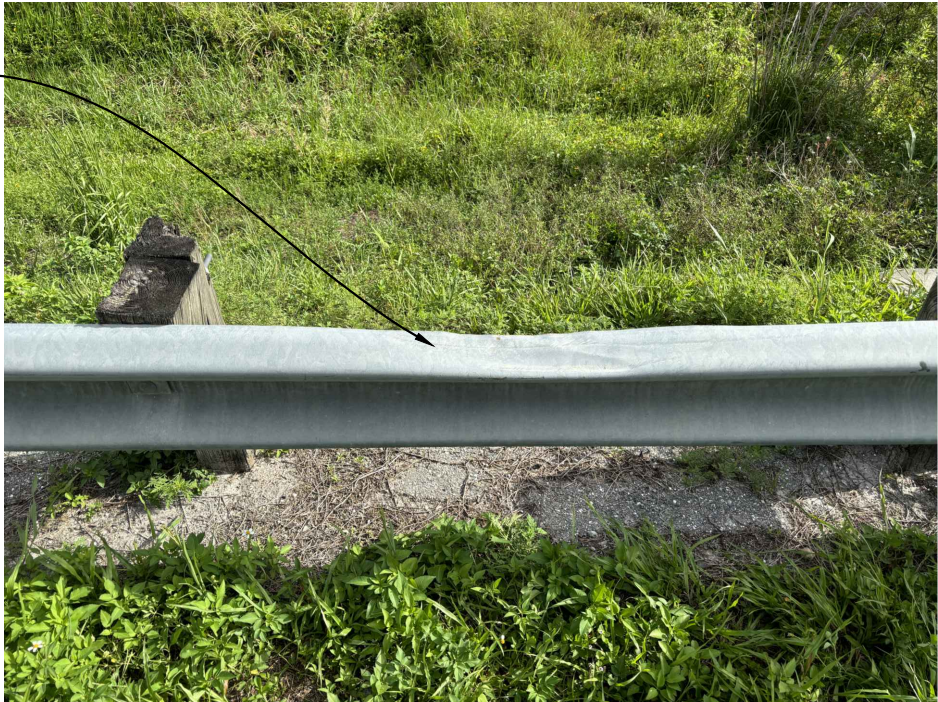
PHOTO 12 - BEGIN, LEFT GUARDRAIL
