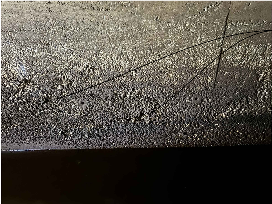
PHOTO 8 - TYPICAL SIDE WALLS (CLOSEUP)
