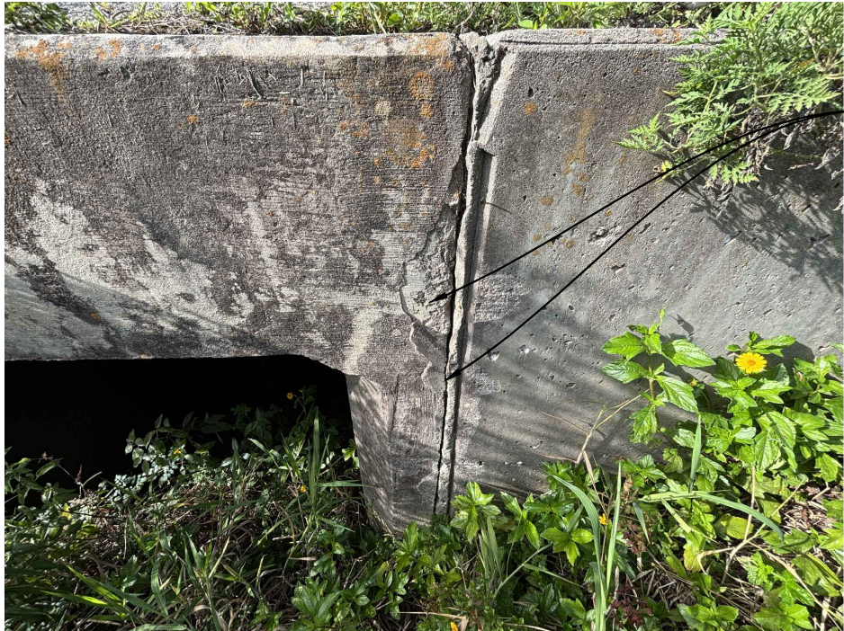
PHOTO 3 - TYPICAL HEADWALL/WINGWALL JOINTS
