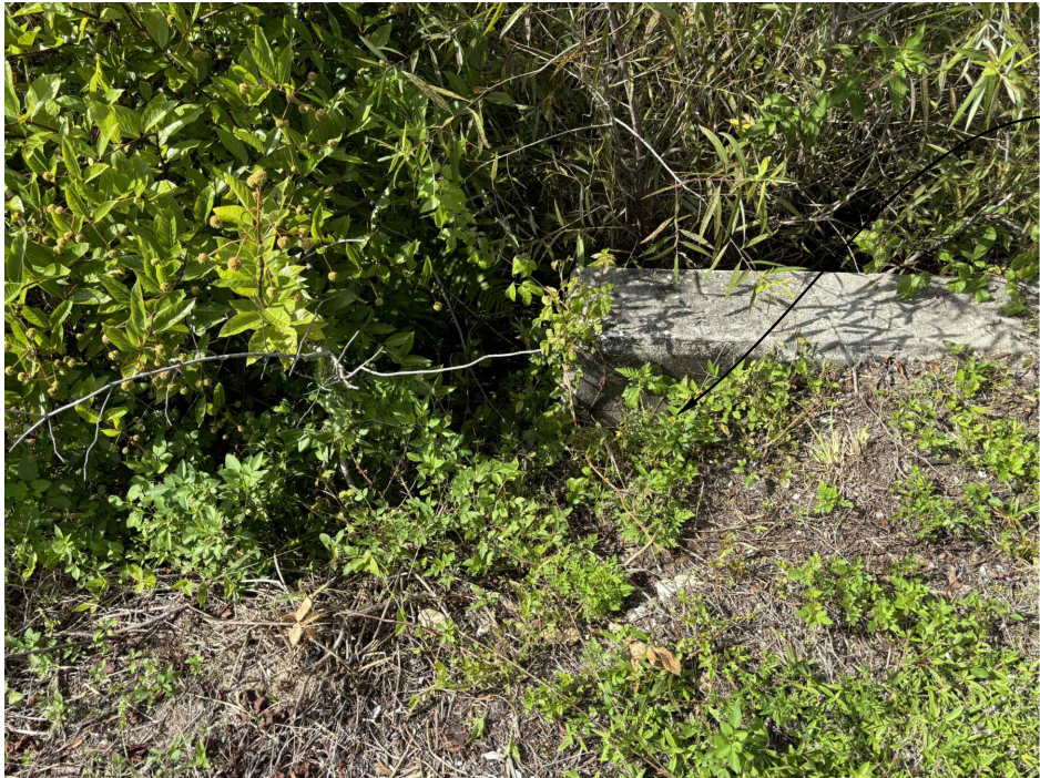
PHOTO 8 - END, RIGHT WINGWALL
