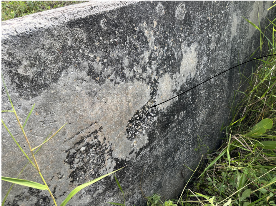
PHOTO 5 - BEGIN, RIGHT WINGWALL
