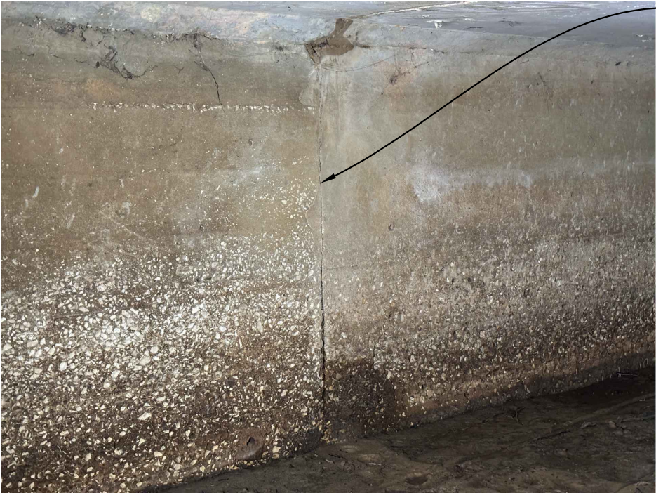
PHOTO 18 - TYPICAL WIDENING JOINTS
