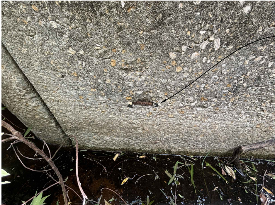
PHOTO 7 - END, RIGHT HEADWALL
