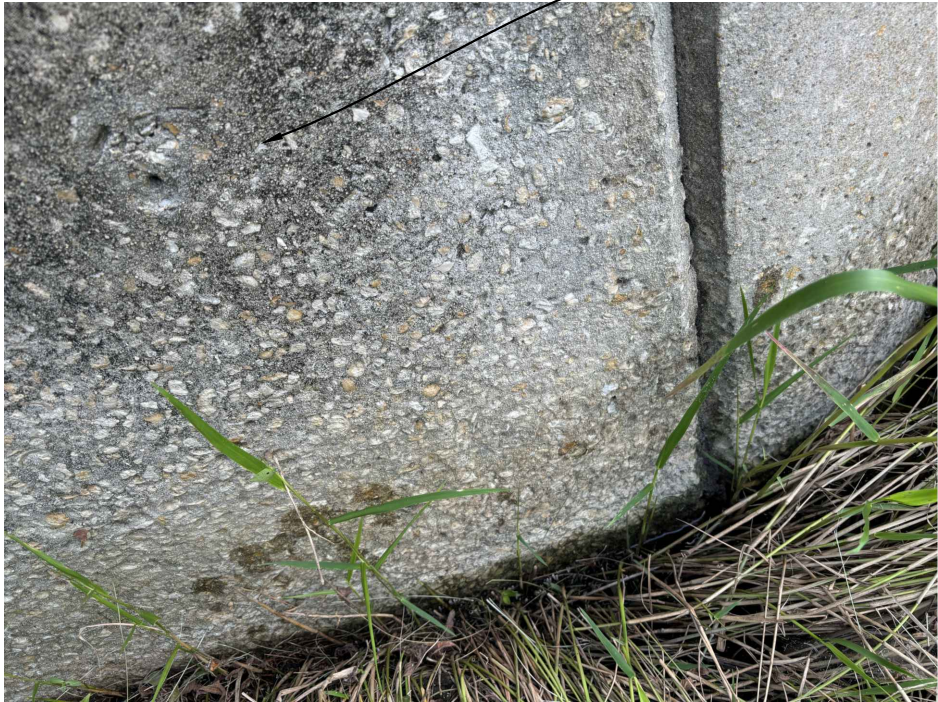
PHOTO 6 - BEGIN, RIGHT WINGWALL
