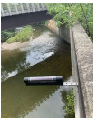
Drilled into Concrete
