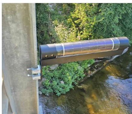
Strapped to bridge/crossing
