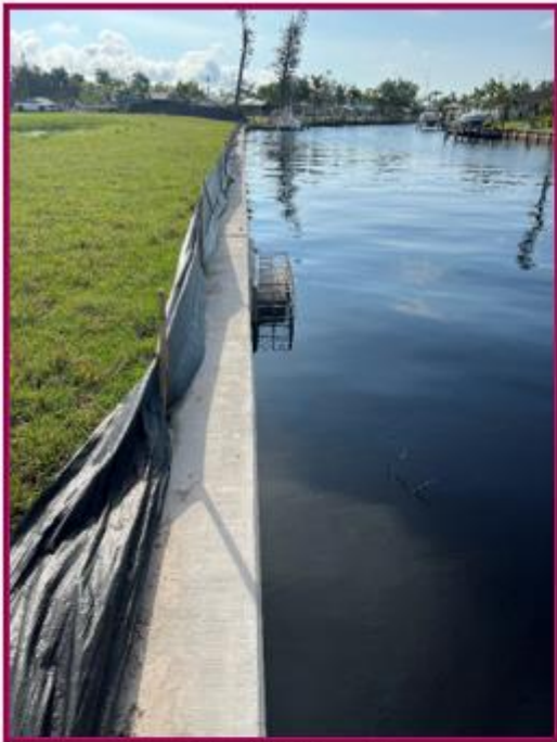
Lister Park Seawall
