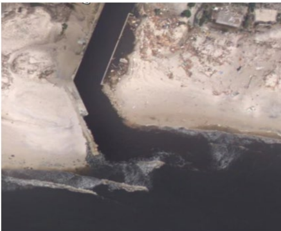
Figure 8. Mexico Beach Jetty and Canal Opening
