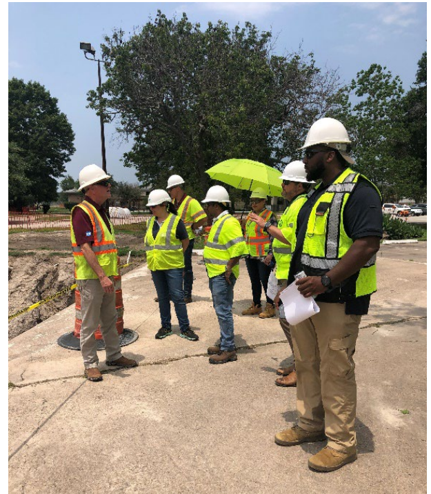
Figure 4. The AtkinsRéalis team performed a site inspection for a large-scale infrastructure resilience project with state representatives for the City of Houston.
