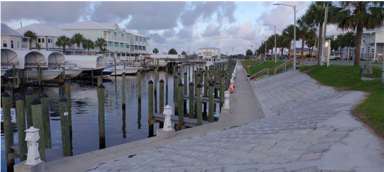
Figure 14. Mexico Beach Marina hardening with armor stone.
