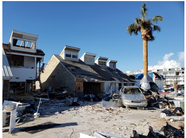
Figure 10. Devastation from Hurricane Michael resulted in damage to 80 percent of infrastructure for the City of Mexico Beach.
