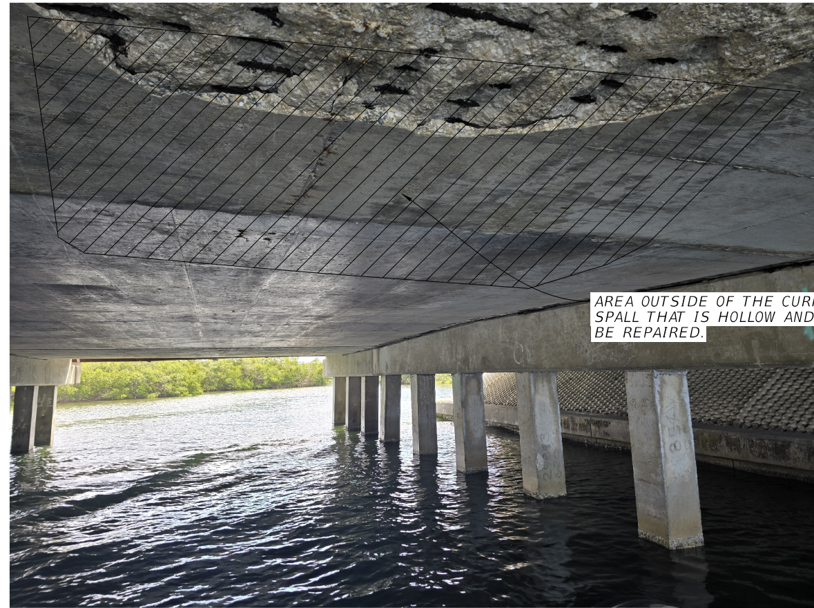
PHOTO 2 - SPAN 2 WEST SPALL
