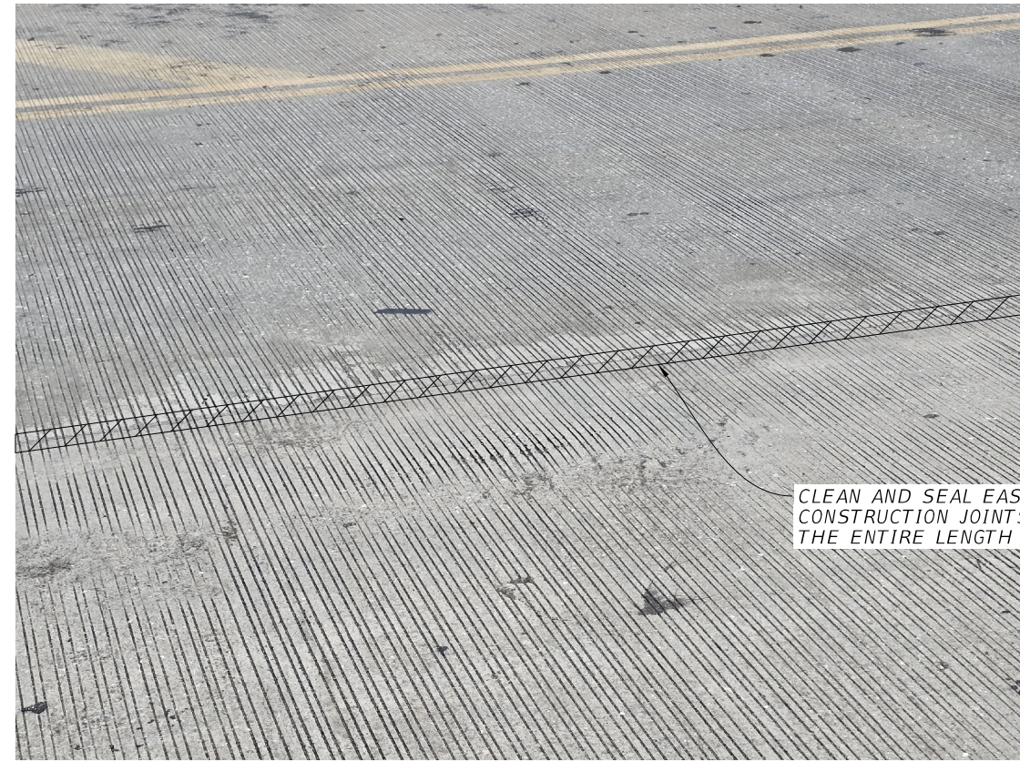
PHOTO 6 - EAST CONSTRUCTION JOINT
