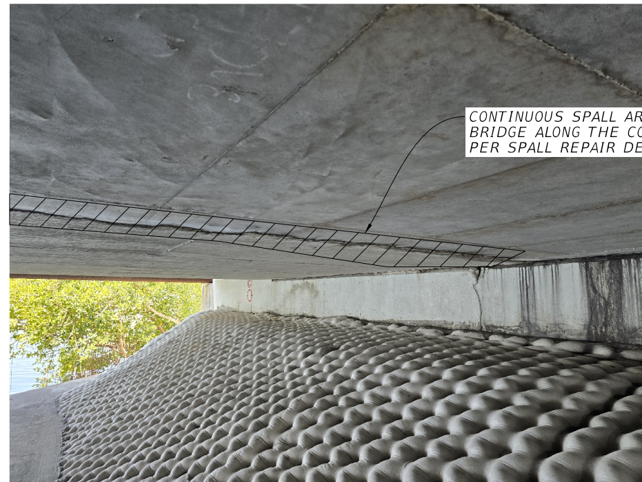
PHOTO 4 - WEST SPALL ALONG CONSTRUCTION JOINT
