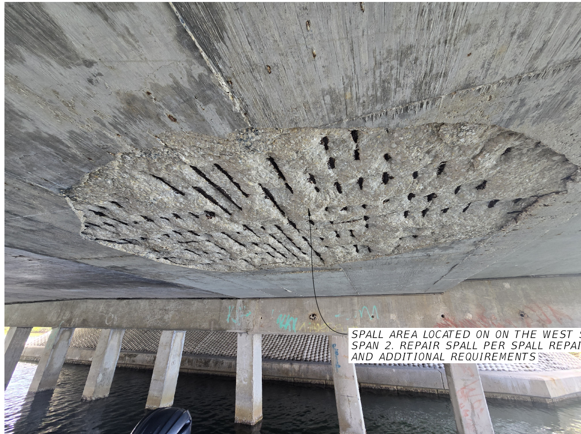
PHOTO 1 - SPAN 2 WEST SPALL
