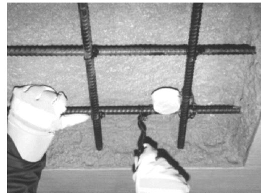
TYPE 1 EMBEDDED GALVANIC ANODE INSTALLATION
