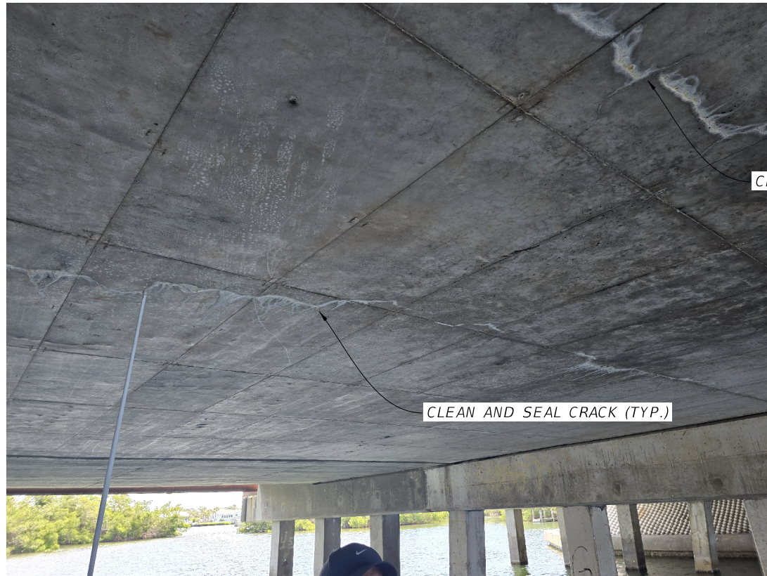
PHOTO 5 - SPAN 3 CRACKS
