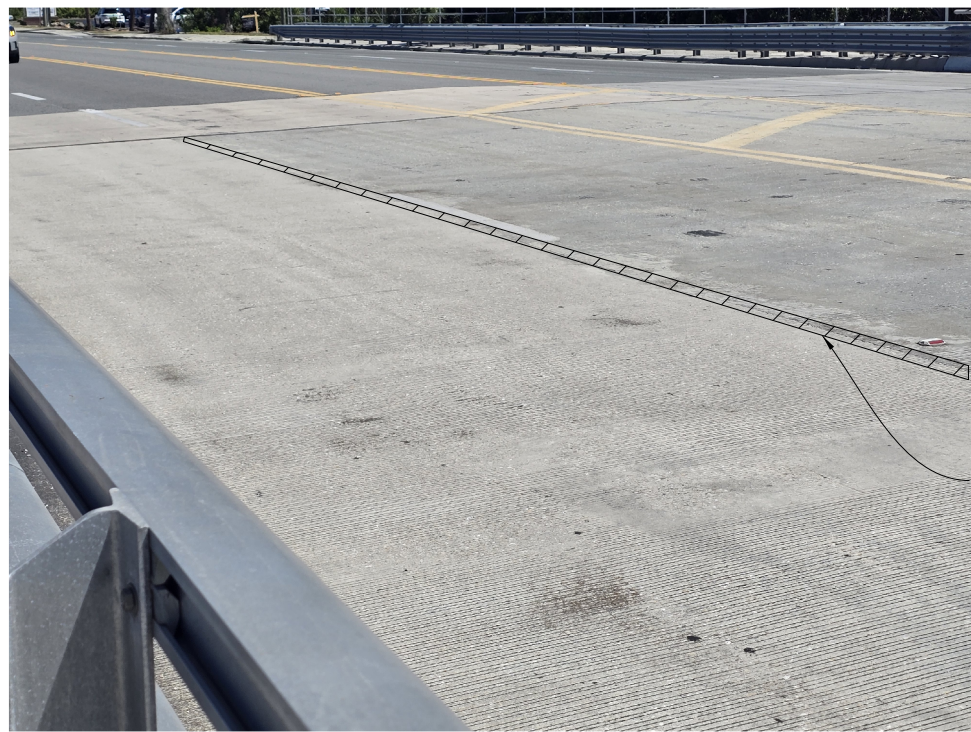
PHOTO 7 - EAST CONSTRUCTION JOINT
