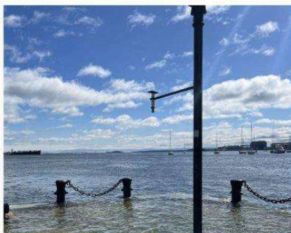
Ultrasonic sensor detecting flooding at Long Wharf Pier in Boston, MA
