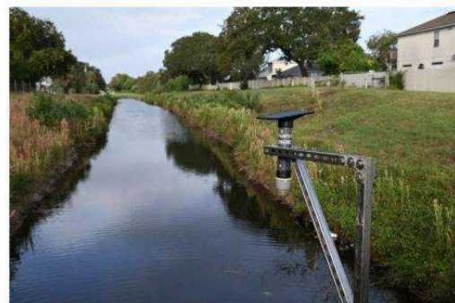
Radar sensor deployed for canal monitoring by Florida DOT
