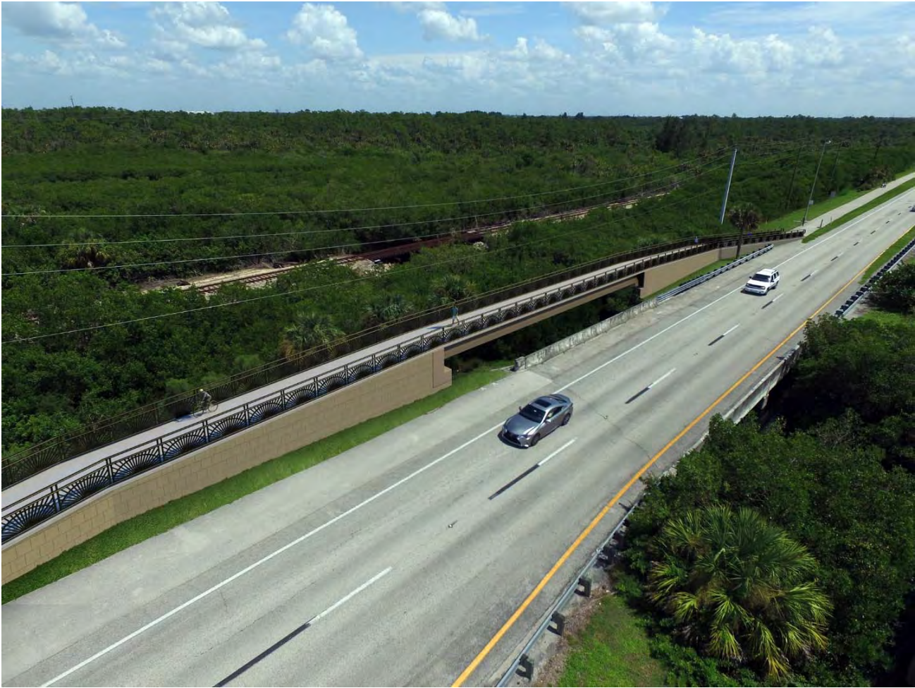
Figure 8: A rendering provided courtesy of the City of Punta Gorda, produced by Agenor & Campbell Structural Engineers.
