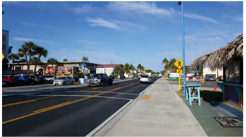
Figure 2: A Complete Street in Fort Myers Beach along Estero Boulevard, a commercial corridor within the Town. Key elements of this complete street include safe, comfortable, and signaled pedestrian mid-block crossings to access destinations, local transit, and speeds suitable to the context of the place.
