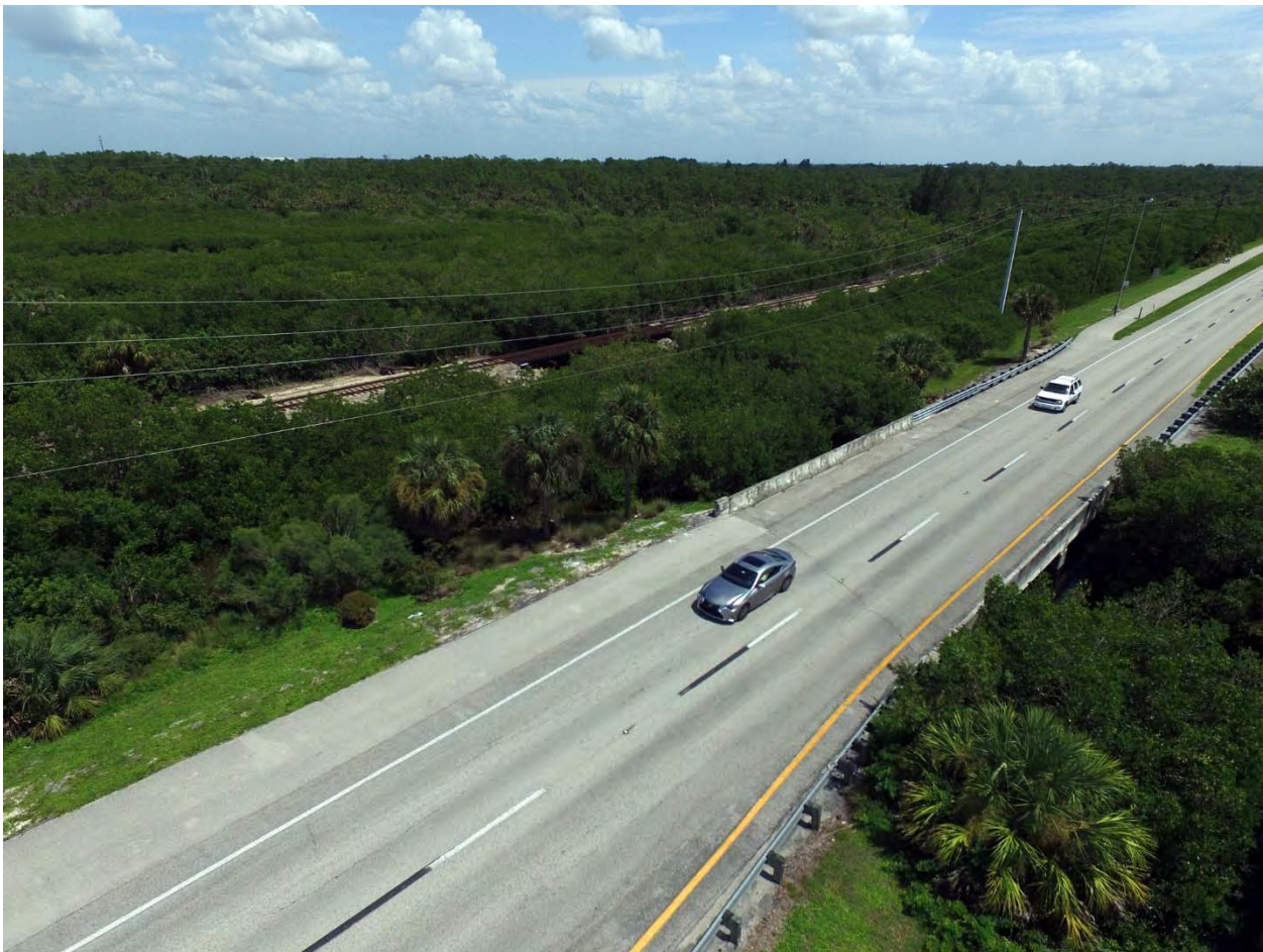
Figure 7: Photo of the US 41 South Trail in Punta Gorda where a gap exists between two segments of existing trail. Photo provided courtesy of the City of Punta Gorda.
