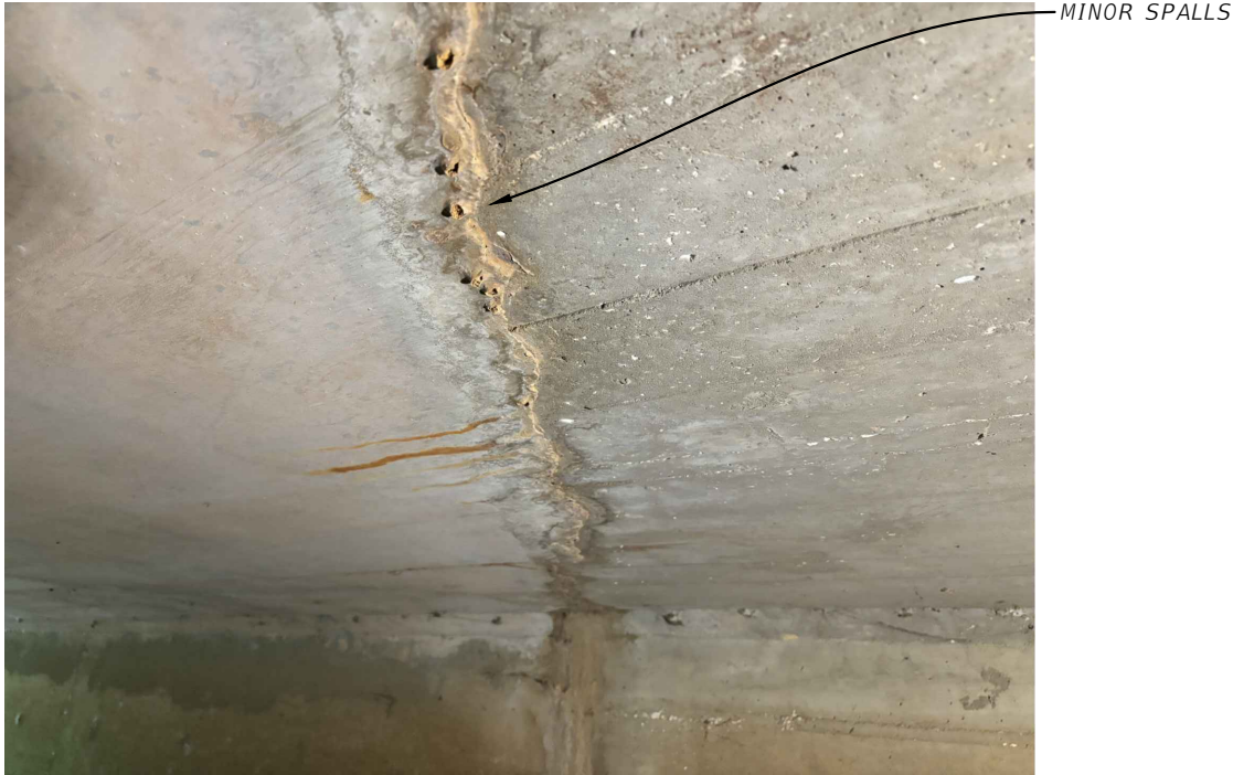
PHOTO 14 - CELL 2, CEILING, RIGHT WIDENING JOINT
