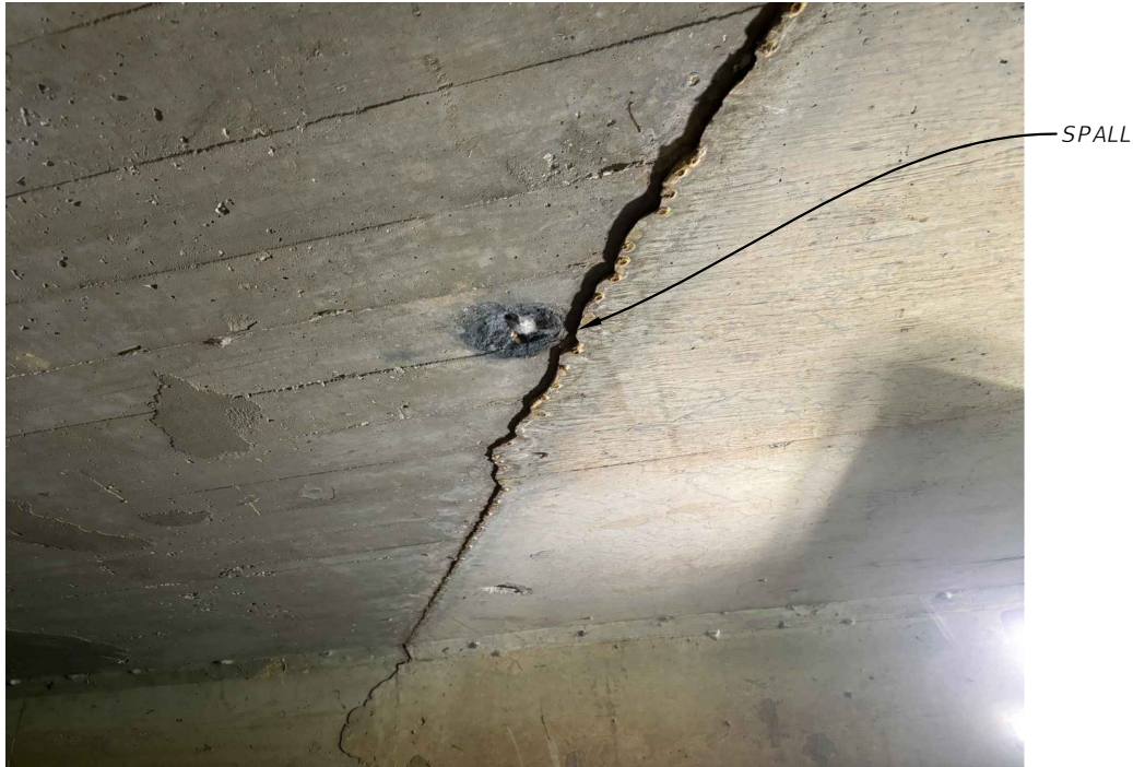
PHOTO 15 - CELL 2, CEILING, LEFT WIDENING JOINT
