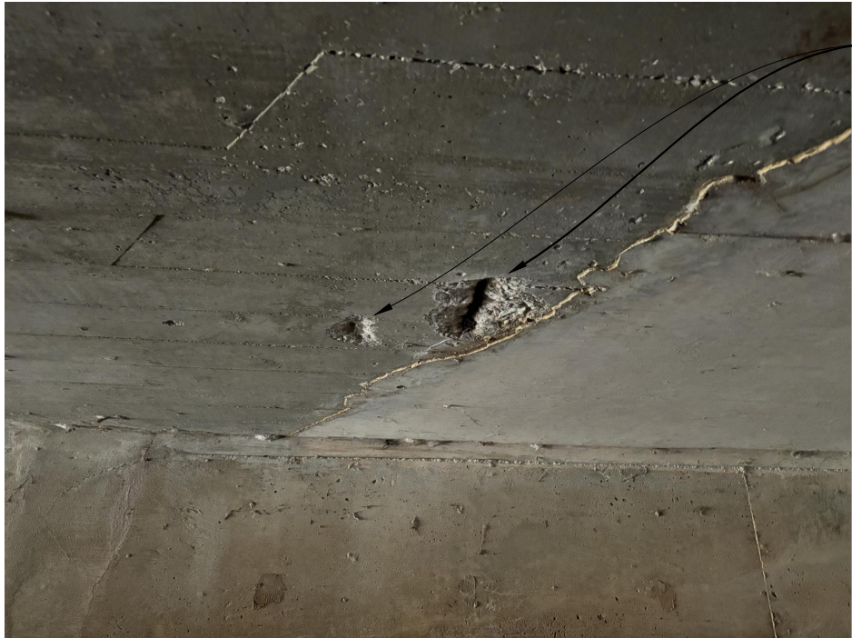
PHOTO 17 - CELL 3, CEILING, RIGHT WIDENING JOINT
