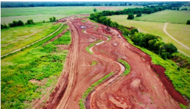
Aerial view of stream, post-construction
