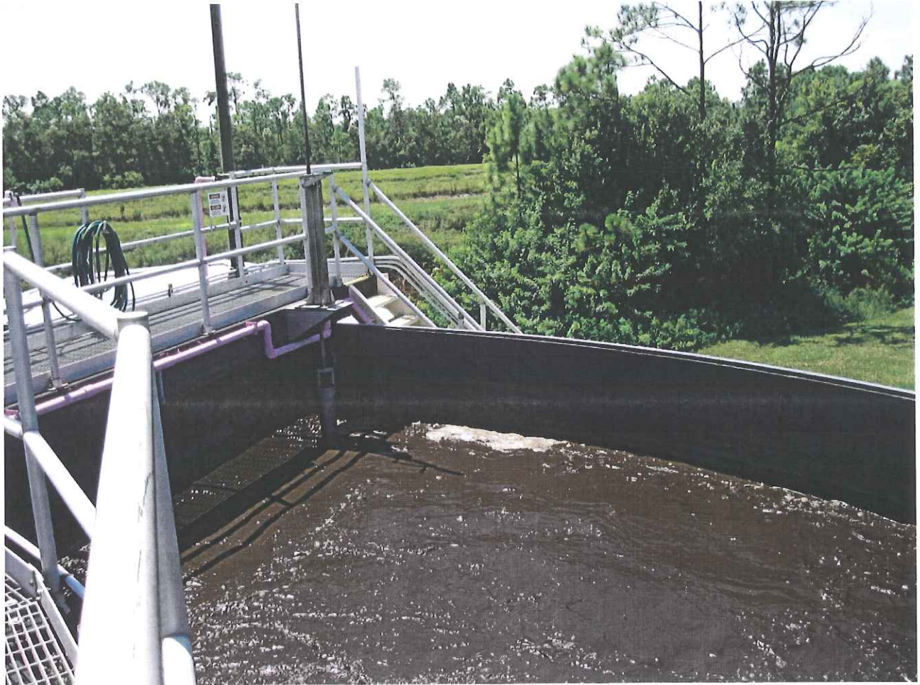
Figure 7- Aerobic Digester
