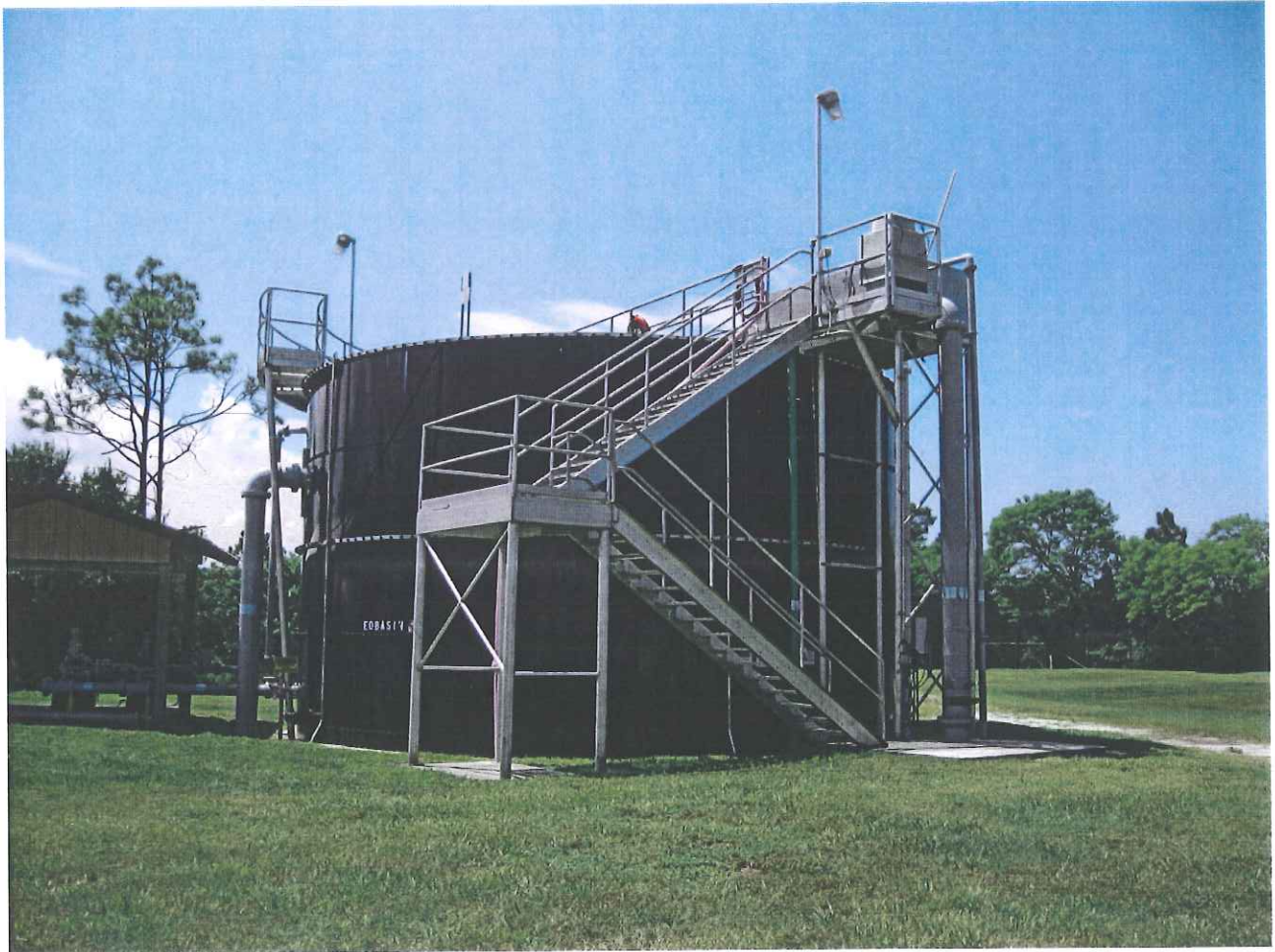
Figure 3- Flow Equalization
