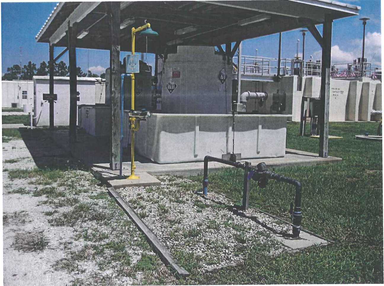
Figure 11- Sodium Hypochlorite Storage
