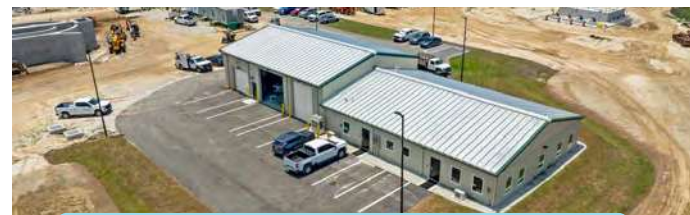
Town & Country Utilities (TCU) Maintenance Building
