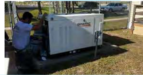
CC Public Works Tranfer System Replacement
