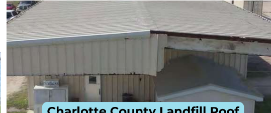
Charlotte County Landfill Roof Repair
