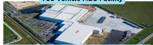
Cheney Brothers Inc Distribution Warehouse Punta Gorda
