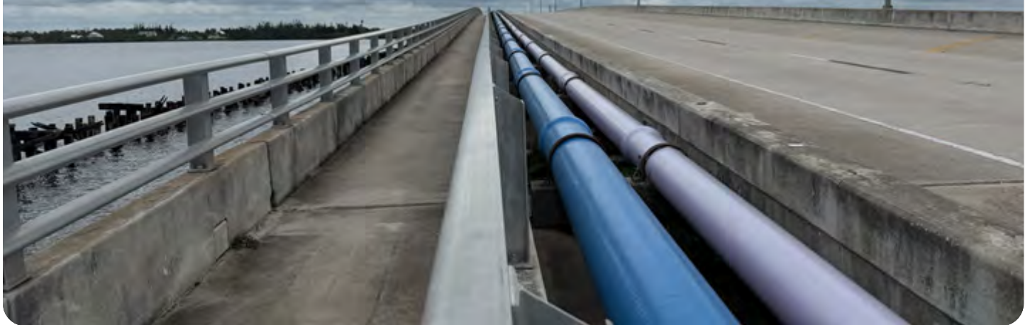
Figure 1: Existing Westbound SR 776 Bridge Looking North Across the Myakka River
