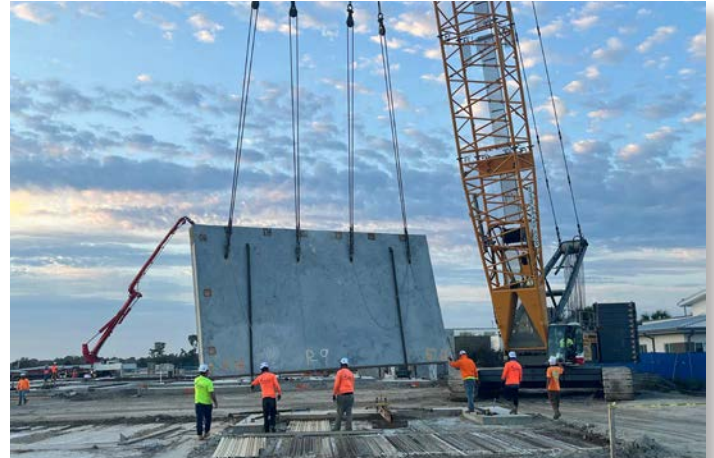
TILT-WALL CONSTRUCTION IN PROGRESS
