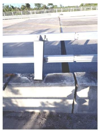
Spall at Bullet Railing Anchorage (Approach Slab Traffic Railing spall shown, Bridge Traffic Railing spall similar)
