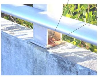
TYPICAL BULLET RAILING ANCHOR CLEANING DETAIL
