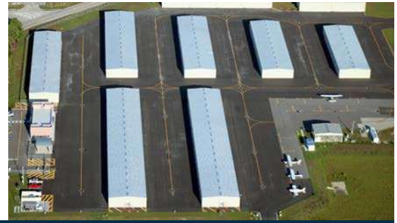
PAGE FIELD SOUTH QUAD HANGARS & RAMPS
