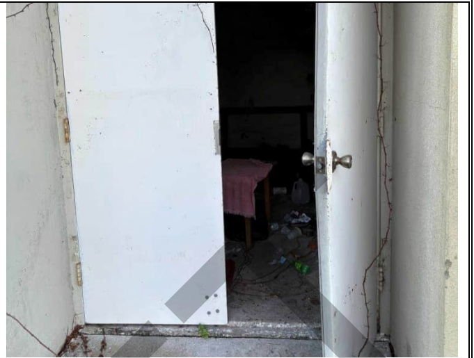
Photo 2: Entrance to one of the locked doors.
