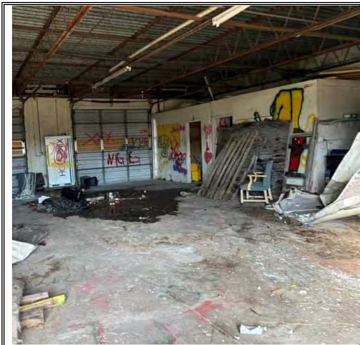
Photo 5: Inside the garage area.
