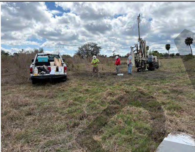
Photo 11: Location of SB-15/TMW-4.
