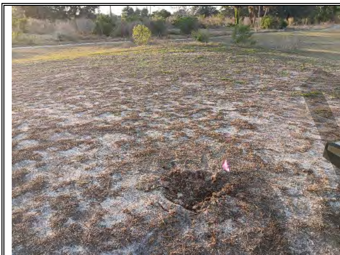
Photo 23: TMW-6 pulled out and backfilled.
