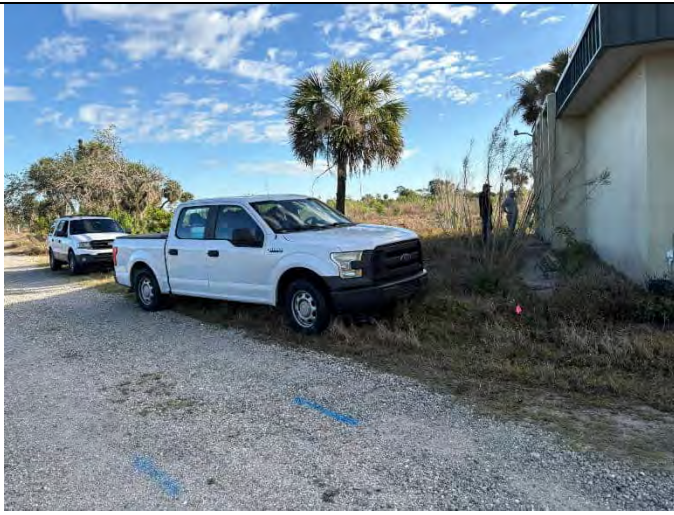
Photo 1: General site photo for Area 1-Maintenance Building.
