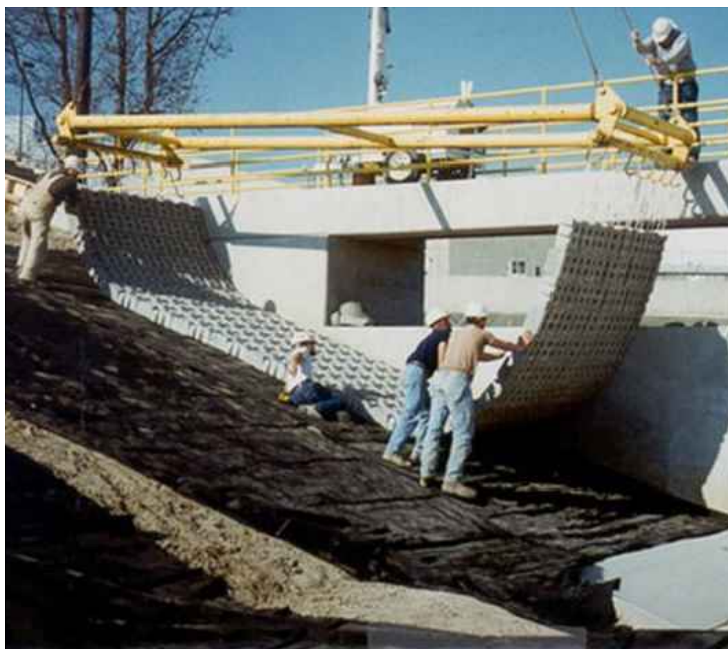
ARMORFLEX INSTALLATION
