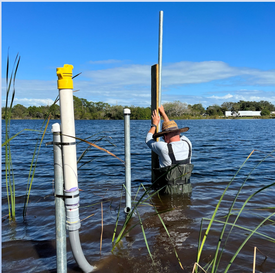
Thomas Prevratil installing equipment at Indrio Savannah Preserve
