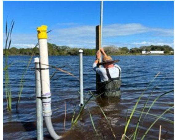
Building a water level sensor station in Lake Indrio
