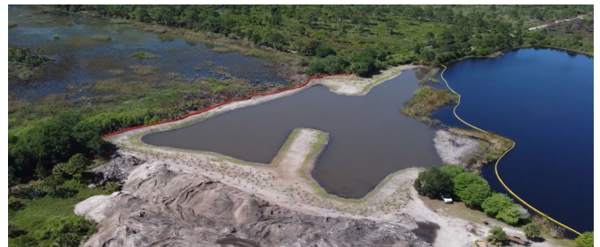
Indrio Savannahs Wet pond and flow features under construction
