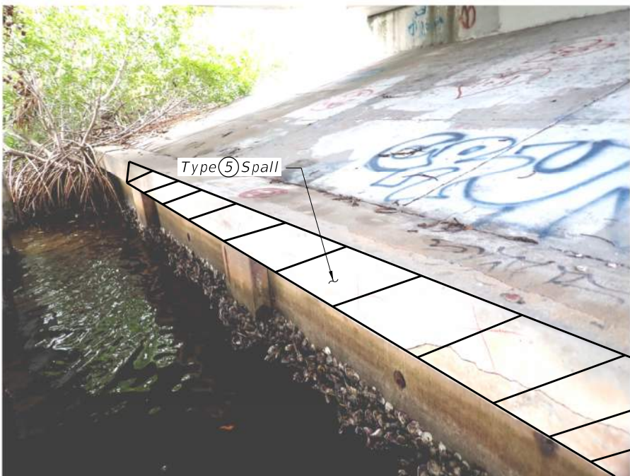
Bulkhead Wall Cap (West Bulkhead Wall shown)
