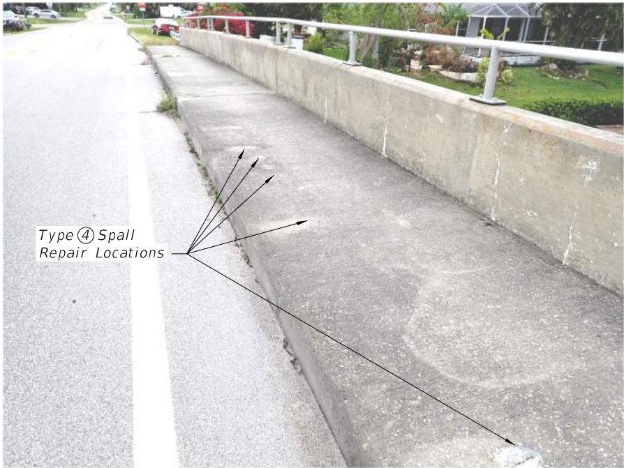
Traffic Railing and Sidewalk
