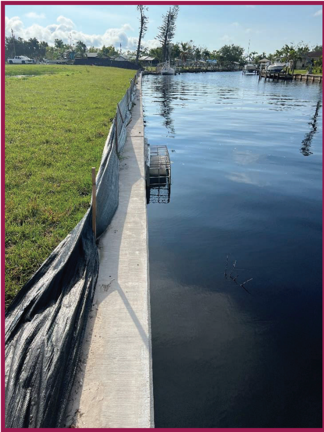
Lister Park Seawall
